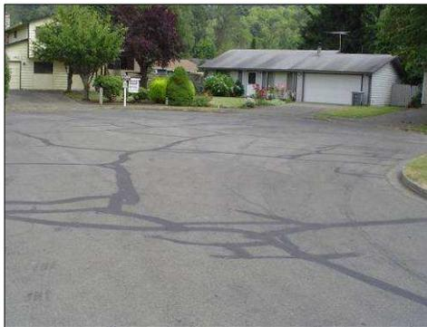
20<sup>th</sup> St NE after crackseal
